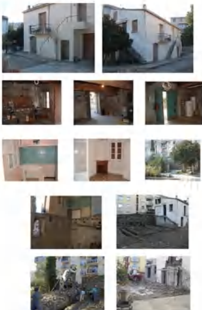
French house renovation, 2007–2008
