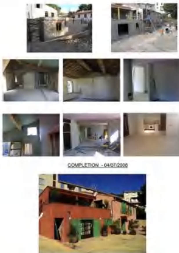
French house renovation, 2007–2008
